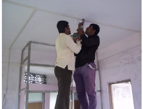
Trainees of Electrician Trade at Extension Centre - Mangaon
