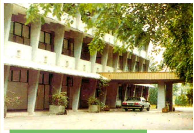
CPSC Building in Singapore (1973-1986)
