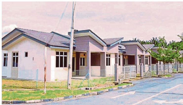
Figure 2: Rumah SelangorKu using IBS System
